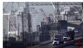
Photos: Terminal Island Freeway
